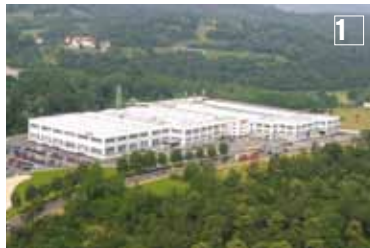
1 Factory - Carpeneda 1 Via Provinciale, 49 25079 Carpeneda di Vobarno (Brescia) Italy Total surface area m 2 131,000 Covered surface area m 2 32,500
